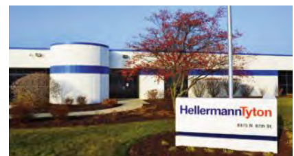
Offices and Manufacturing 87th Street, Milwaukee, WI
