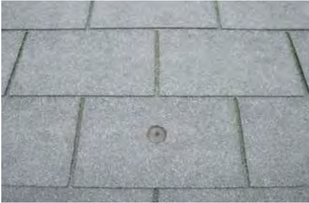
THREE TAB shingle roof
