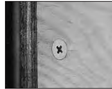
Plywood to steel or wood studs.
