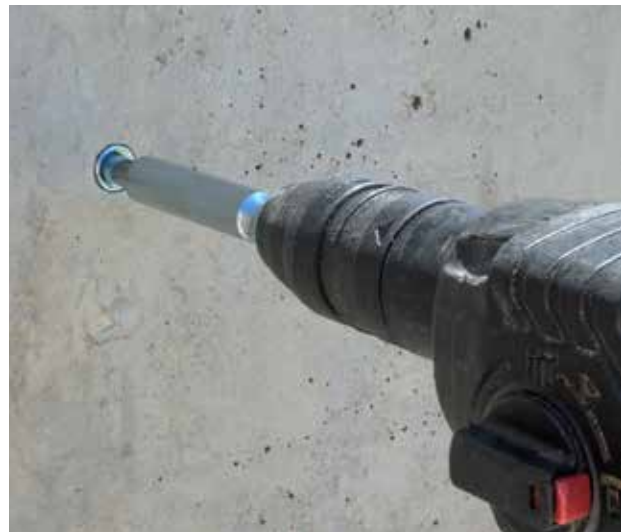
Anchor being set with SDS setting tool.
