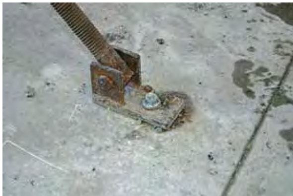
The Titen HD® screw anchor 3/4" x 6" and 3/4" x 7" (models THDT75600H and THD75700H) have a 1" section under the head that is unthreaded to allow installation into tilt-up wall braces.
