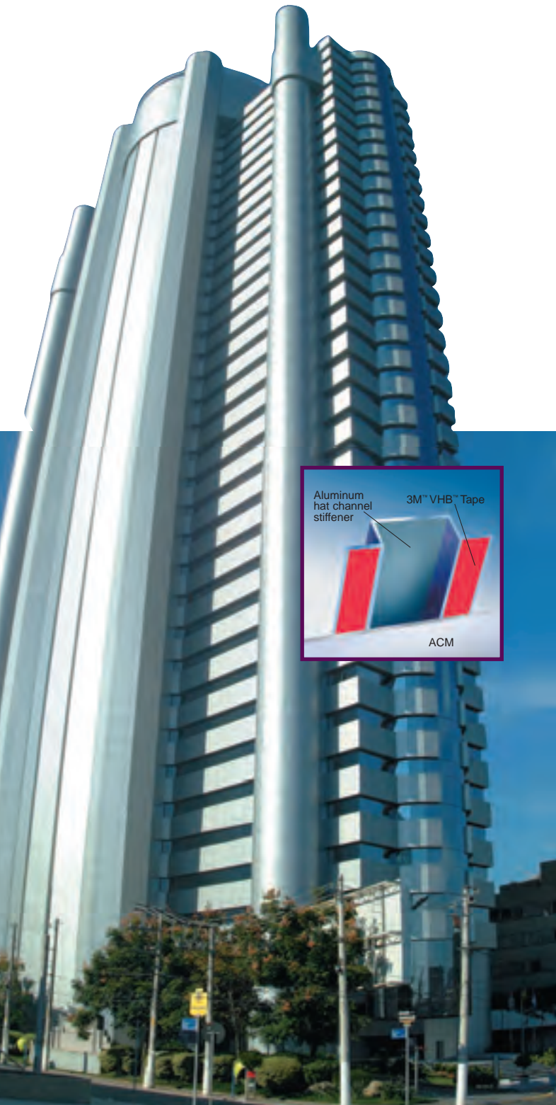
Plaza Centenário, Sao Paulo, Brazil Architect: Carlos Bratke, 1995 Aluminum stiffeners bonded to ACM panels.
