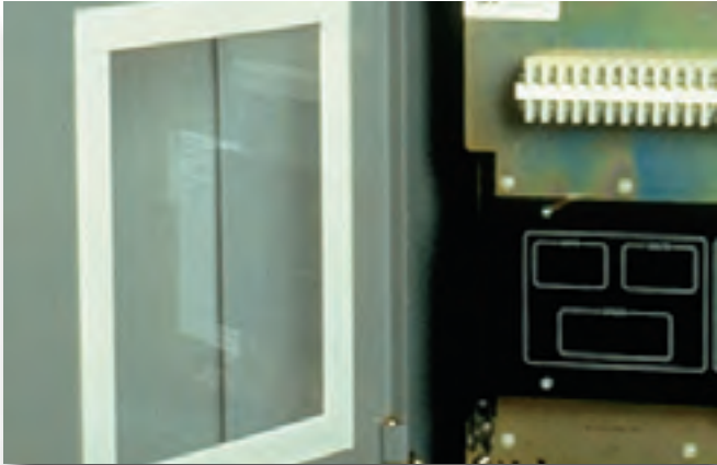
Bond and seal polycarbonate viewing window into the door of a process control system.
